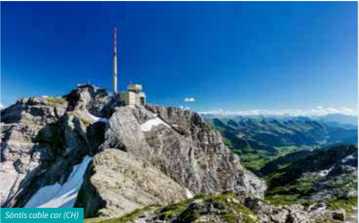
Säntis cable car (CH)
